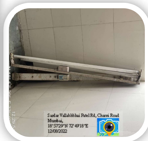
Replacing with led lights
