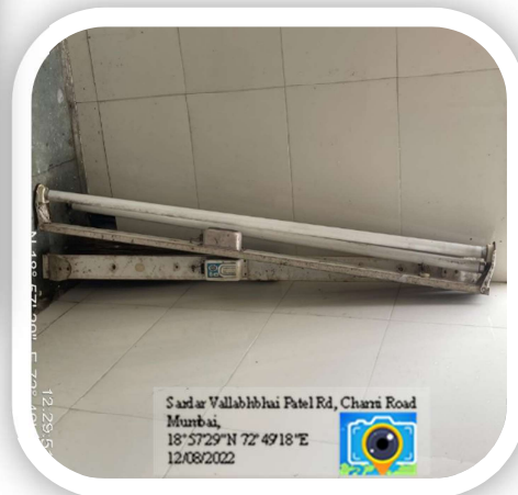
Replacing with led lights
