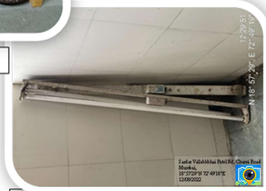
Replacing with led lights
